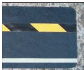
Luminous stripe & hazard warning stripe
