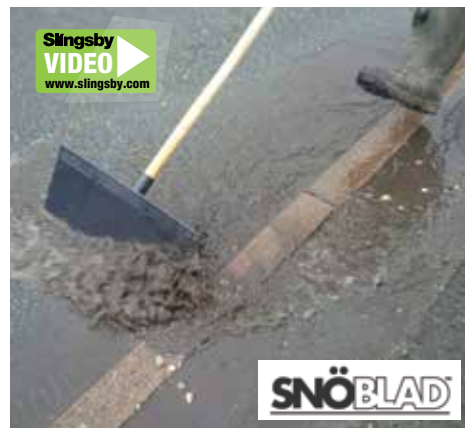
Direct rain water into drains
