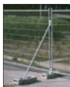
Fence stabiliser + concrete foot
